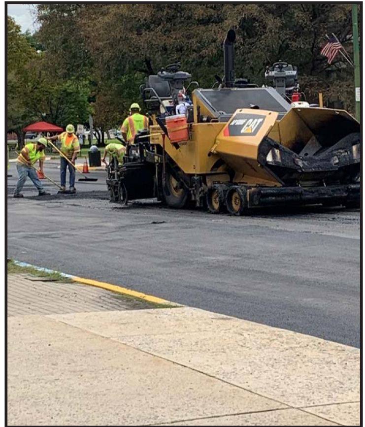
The paving of Delaware Avenue's broad expanse required application of black top in four equally spaced stages along the entire length of the thoroughfare. Traffic control was a challenge.
