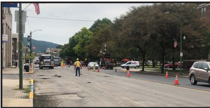
Delaware Avenue is scraped ....
