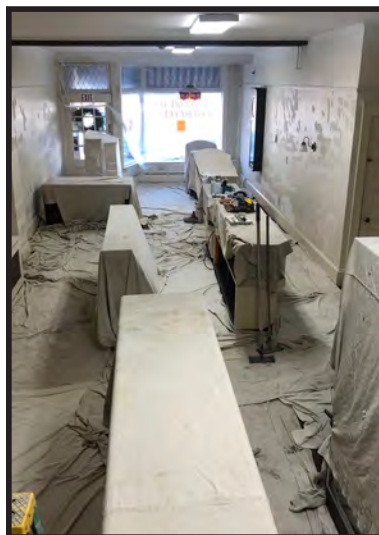
... a fresh coat of paint
